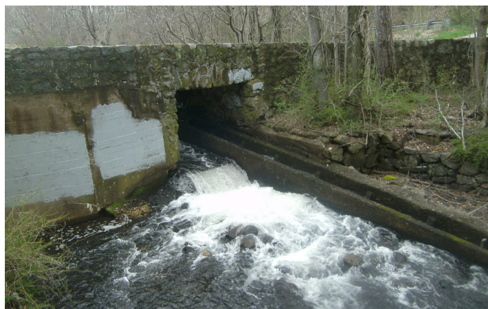
Billington Street Dam prior to removal. Source: Mark Rousseau, MADMF
