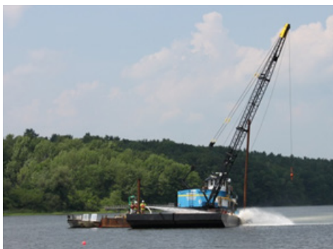
Spreading clamshell by hose and barge. Source: Megan Latour
