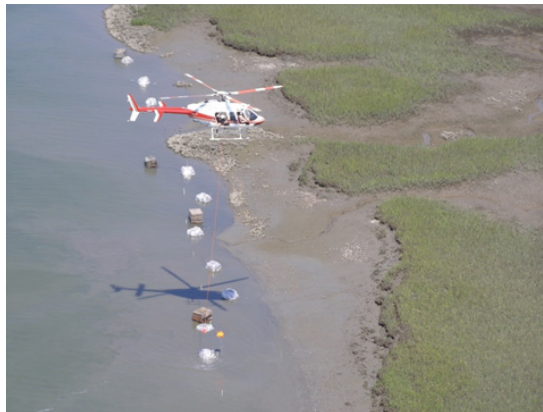
GADNR helicopter transferring shell material to Oyster Creek restoration site. Source: Larry Rogers, GADNR Aviation Division
