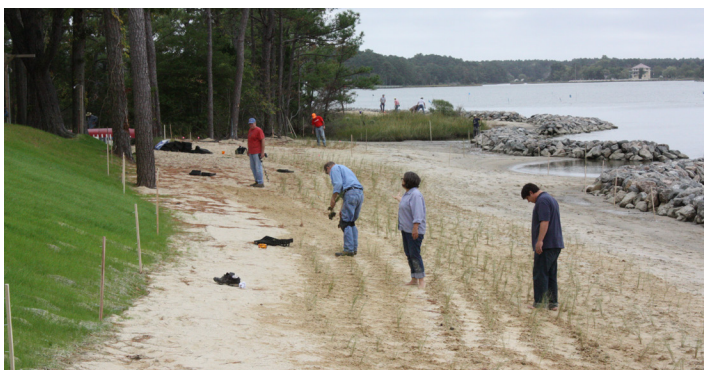
Volunteers planting marsh grasses along newly constructed living shoreline that includes low rock sills protecting a newly graded marsh terrace. Source: Gwynn Crichton
