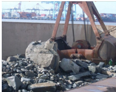
US Army Corps of Engineers harbor deepening project dredge rock. Source: US Army Corps of Engineers
