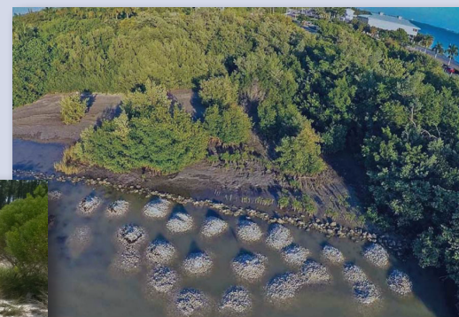
Punta Rassa, Florida after living shoreline installation (above). A living shoreline constructed in Panama City, Florida using plants and oyster shell (left). Photo credit: www.floridalivingshorelines.com .
