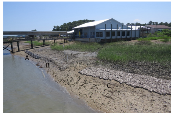
South Carolina DNR deploys (A) oyster castles, (B) concrete-coated crab traps, and (C) bagged shell as living shorelines. Photo credit: SC DNR.
