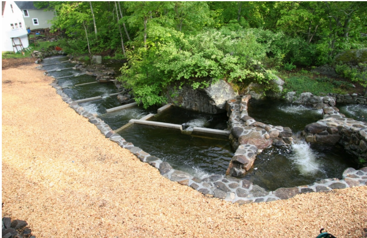
Figure 12. Upper section of the fishway after restoration.
