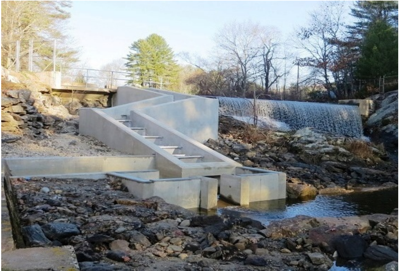
Figure 29. The Nequasset fishway and entrance to the trapping facility after repair in 2014.
