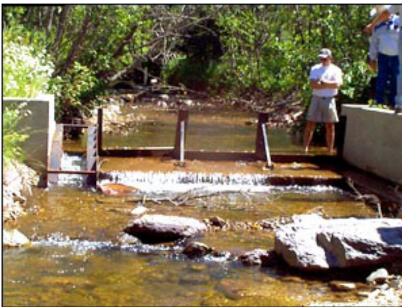
Figure 1. Reconstruction of an irrigation canal with a fish ladder on Chamberlain creek, a tributary stream of the Blackfoot River. Source: U.S. Fish & Wildlife Service ( http://montanapartners.fws.gov/mt5c.htm ).
